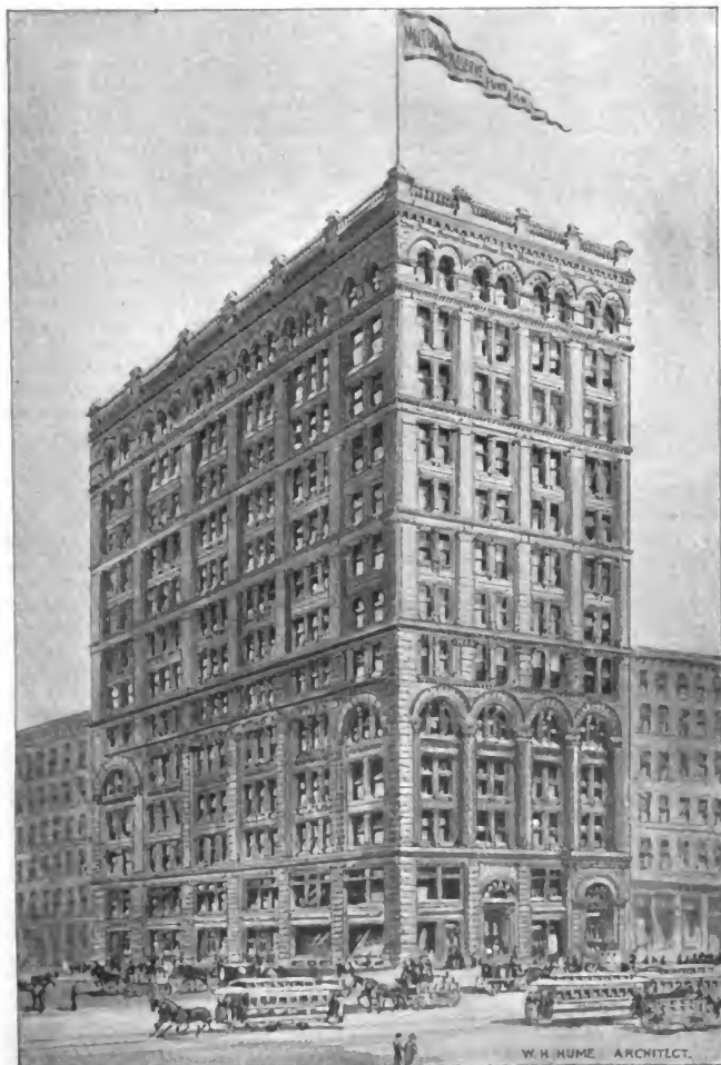
MUTUAL RESERVE FUND LIFE ASSOCIATION. MUTUAL RESERVE BUILDING, BROADWAY, NORTHWEST CORNER OF DUANE STREET.
